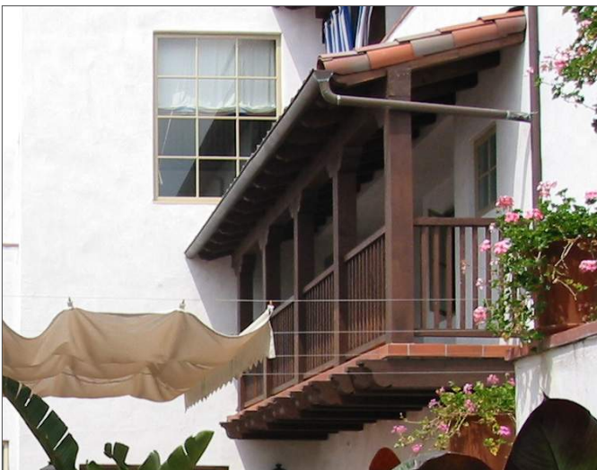
A wood balcony supported by extended beams
