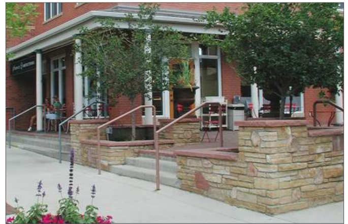
Site walls laid in ashlar pattern.
