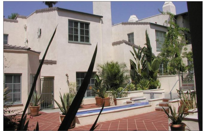
Plaster walls with pre-cast concrete caps.
