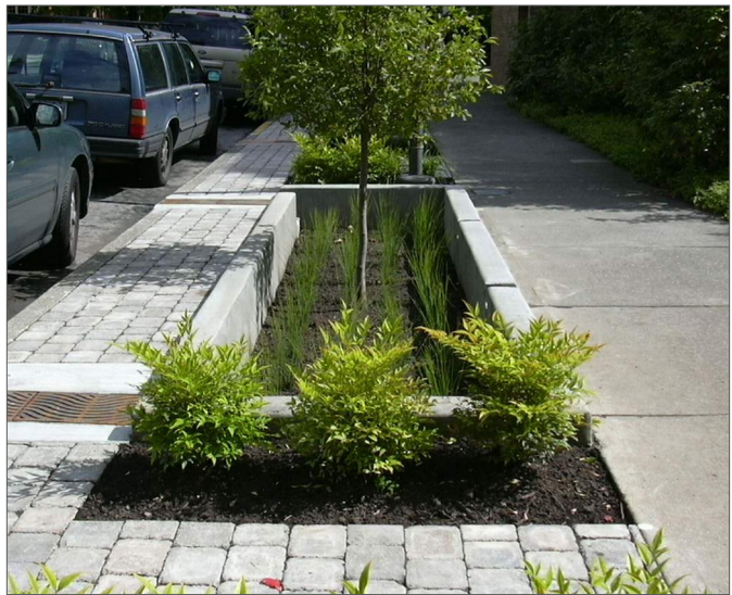
A curbside rain garden collects and filters storm water.
