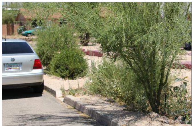
Drainage channels may be cut into street curbface to allow street run-off water to drain into medians, providing biofiltration and wastewater management.
