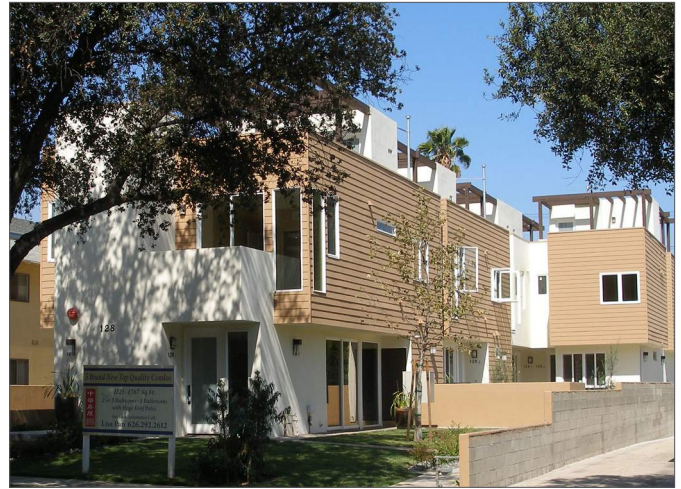
Trellises covering rooftop decks.
