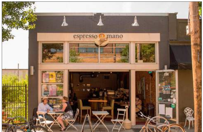
Commercial sectional garage frontage
