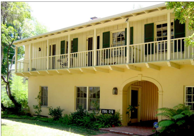
Example of a covered passage.
