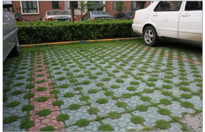
Permeable pavers within a parking area
