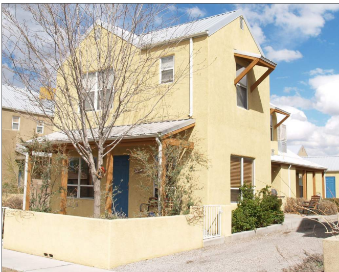
Brackets support a metal window awning.
