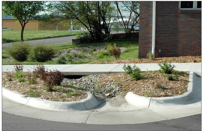
A bulb-out containing a swale with access to street runoff
