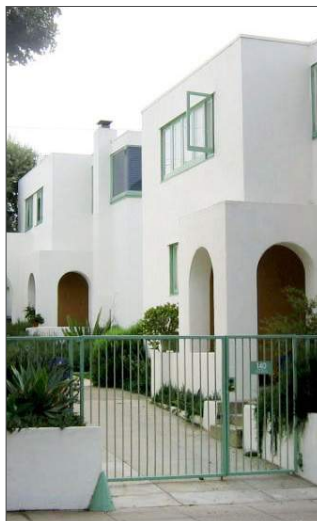
A modern parapet
