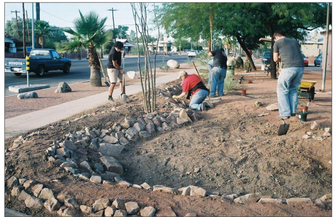
Installation of a desert detention area
