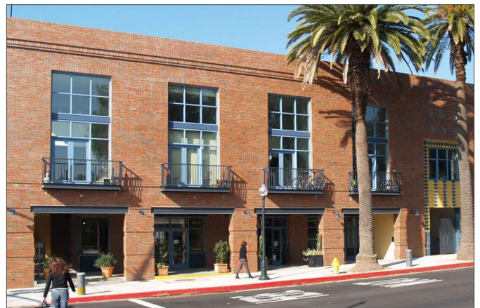
A brick building with an articulated parapet
