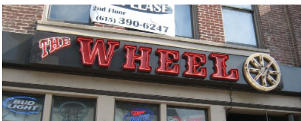
Example of raceway incorporated as sign background
