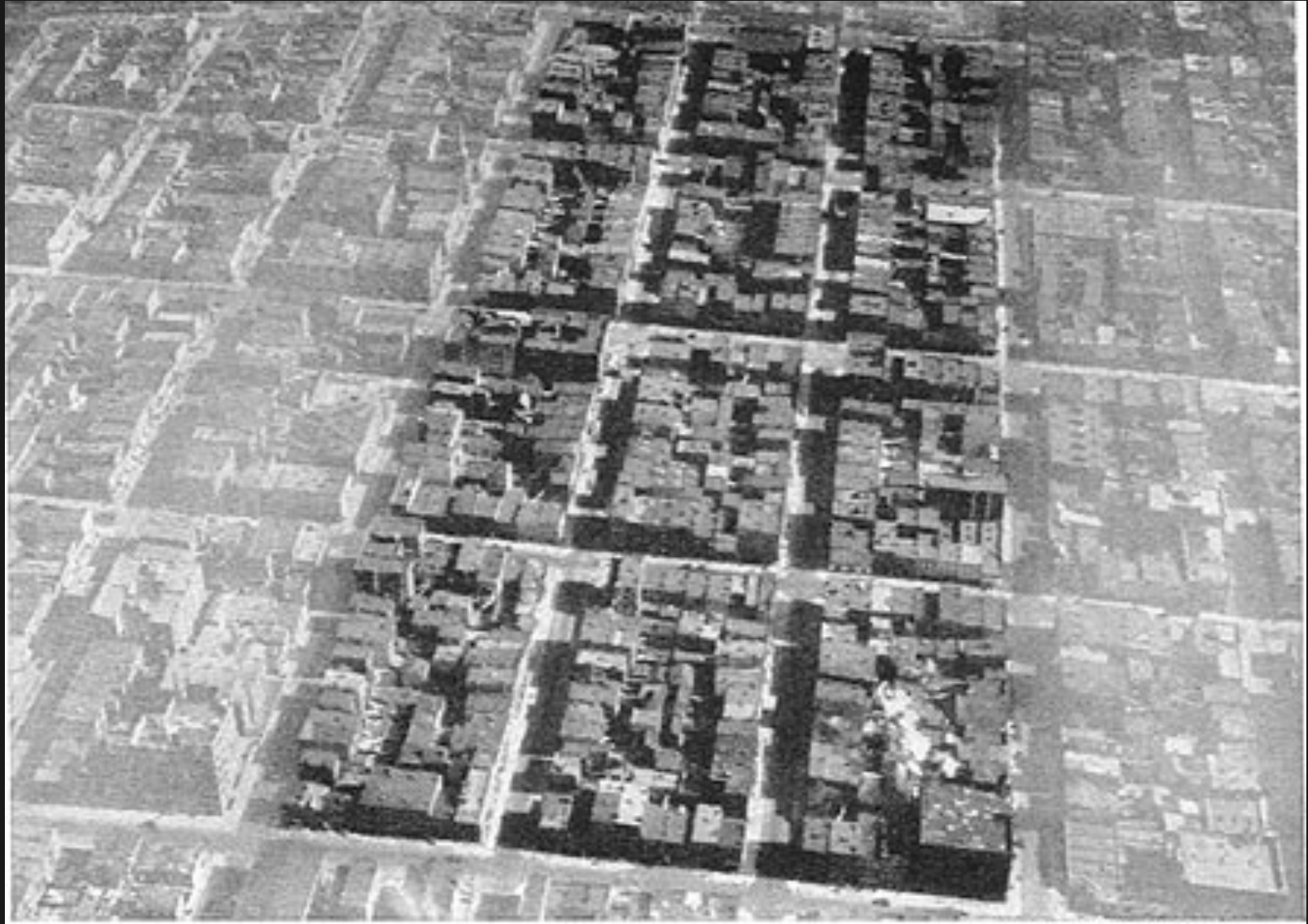
The Original Site
