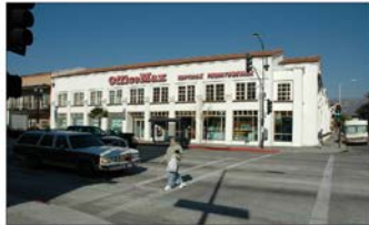
Above: Large Flex Building with parking in rear.
