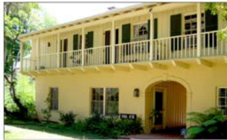
Above: Courtyard Building with front yard facade designed to appear as a large single-family house. Entry to the courtyard is through the zaguan in center of photo.
