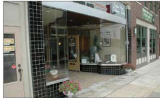
Above: Example of increasing available window space by recessing the entry between flanking shopfronts while remaining visible and connected with the sidewalk.
