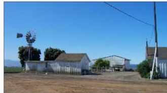
Above: Barn and accessory buildings are organized in support of rural and agricultural activities that emphasize Tehachapi's natural edges.
