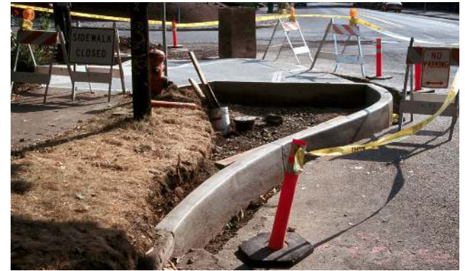
Constructing a Curb Extension, www.pedbikeimages.org/ Dan Burden
