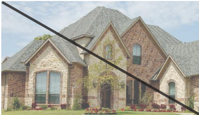
+ Gables and eaves overlap creating confusion rather than a sense of cohesion or evolution of construction.
