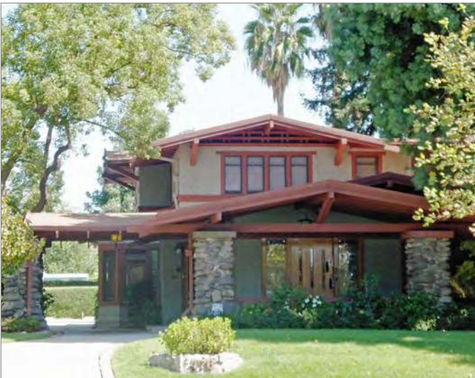
Example: Craftsman bungalow with deep set porch, exposed rafter tails and beams, masonry pier/foundation.
