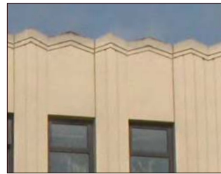
Parapet with serrated coping of plaster
