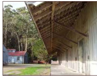
Roof overhang supported by wood struts, decking boards visible
