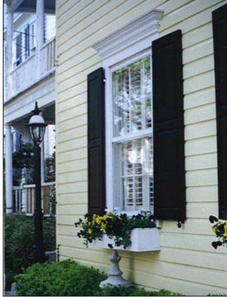
Windows and Doors should be kept simple. Windows should be divided by muntins into multiple panes to provide detail and hold the surface of the façade—rather than the "hole" effect that a large single sheet of glass produces. Specialty windows (oval, octagonal, Palladian, etc.) are encouraged to be one type per building (unit). Windows should be set so that the surface of the panes is recessed at least 2" behind the exterior wall surface (or window surround or shutter).
