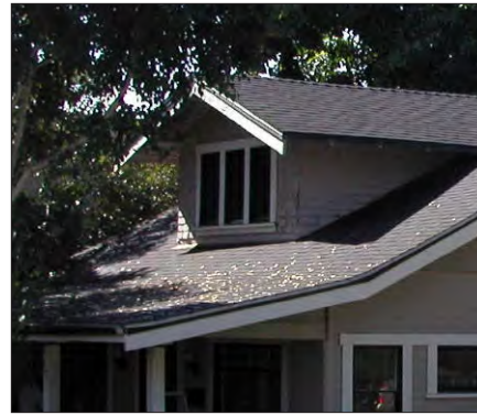
Dormer window with pitched roof
