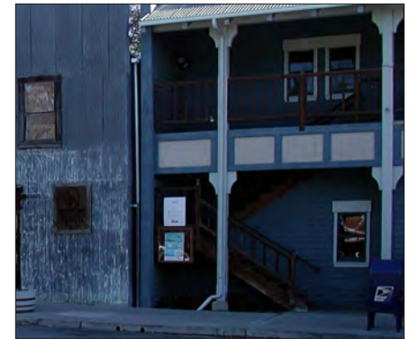
Gutter and downspout along column
