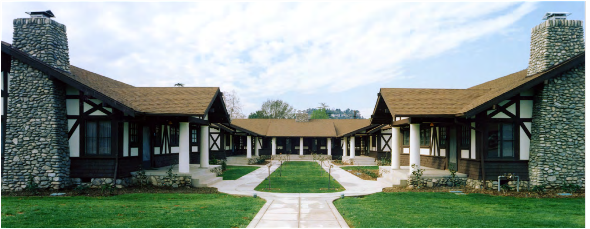
Above: Illustrative Photo: Individual houses fronting a court with the entry porch and/or stoop encroaching into the common space.
