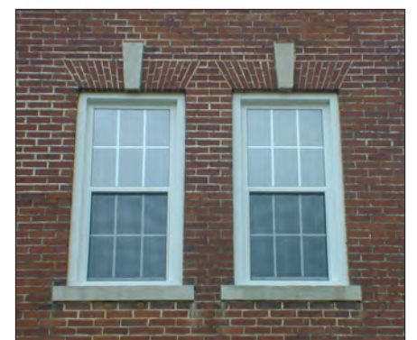
Second-floor windows grouped in pairs
