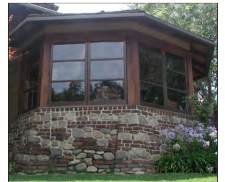
Masonry and stone base
