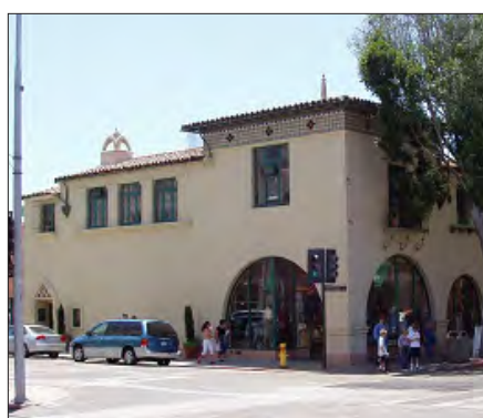
Vertical articulation of corner
