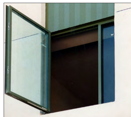
Metal window with metal transom
