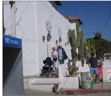
Parapet with flat roof
