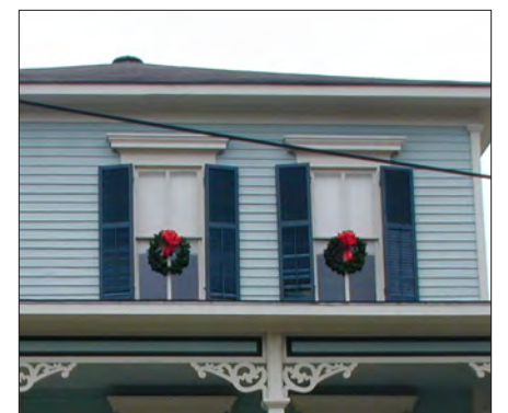
Double-hung windows on second floor
