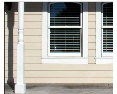
Wood plank siding to grade
