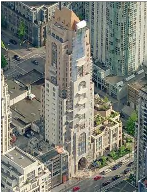
Illustrative Photo: Tower on Podium
