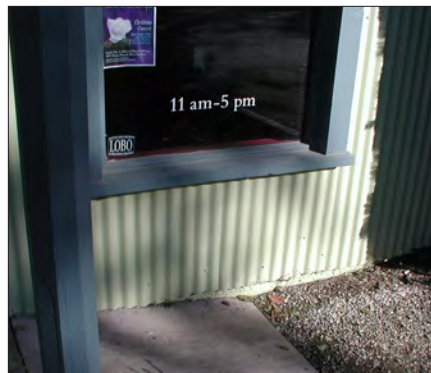
Corrugated siding to grade
