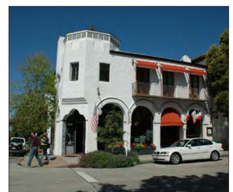
Articulation of corner
