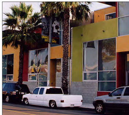
Concrete block base
