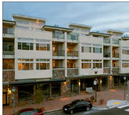
Ground floor as concrete base
