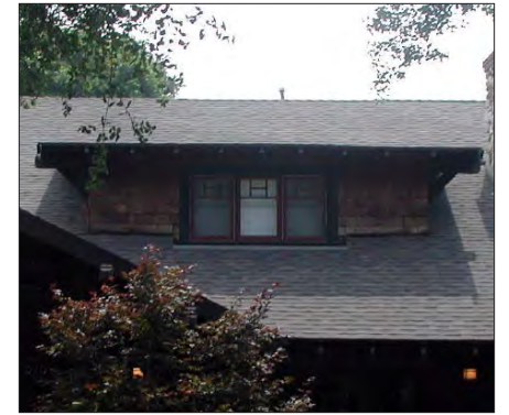
Dormer with "flap-up" roof
