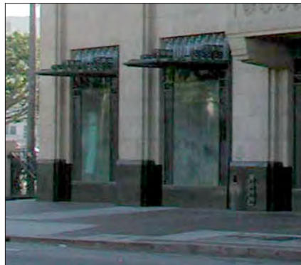
Masonry base and monolithic wall
