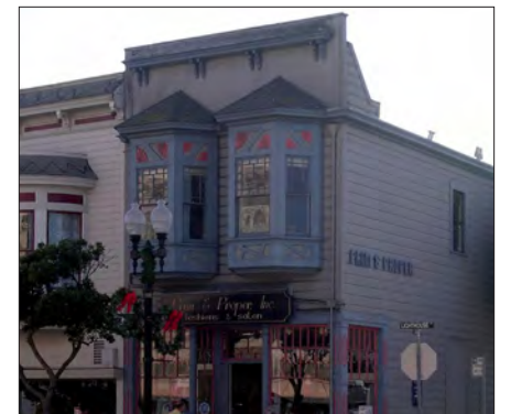
Projecting bay windows
