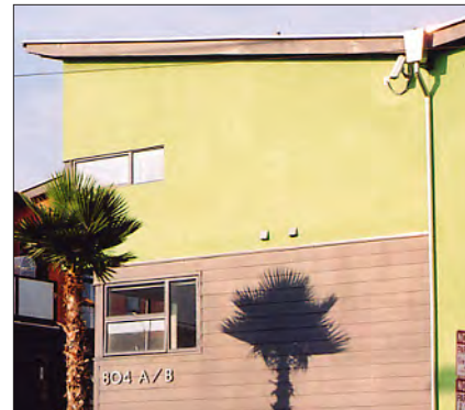
Scupper and downspout
