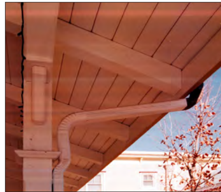
Gutter and downspout
