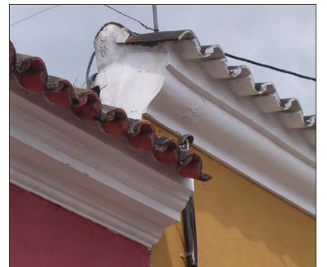
Tile on profiled parapet
