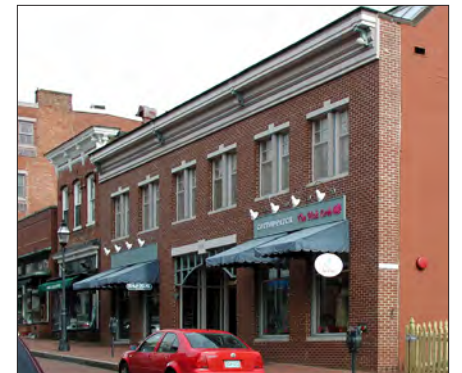
Drainage imbedded in exterior wall
