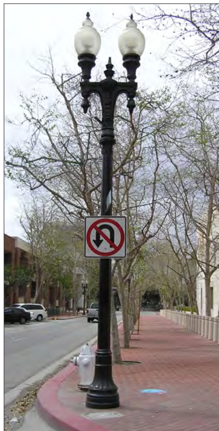
City of Santa Ana Standard Plan 1126 'A' 18' - 0" height to center of lamp refer to City specifications for details
