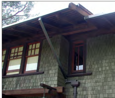
Gutter and downspout
