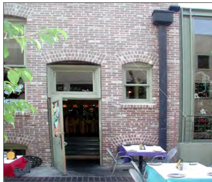
Downspout on back side of building;
