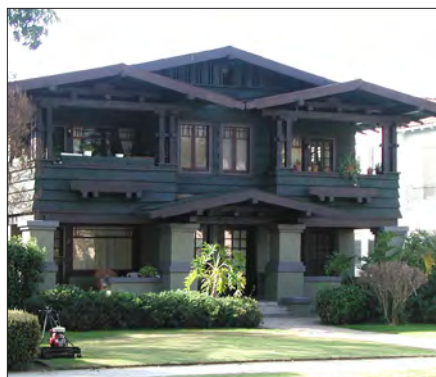
Siding above painted plaster
