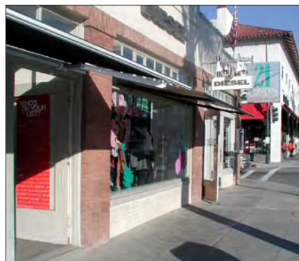
Painted brick transom
