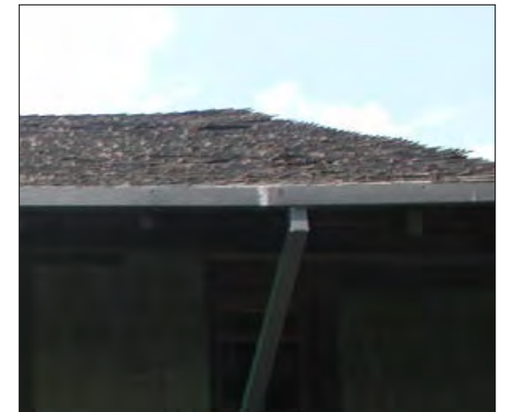
Gutter and downspout
