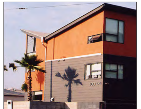
Plaster combined with siding
