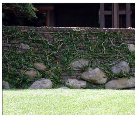
Walls composed of natural materials to blend into landscape
