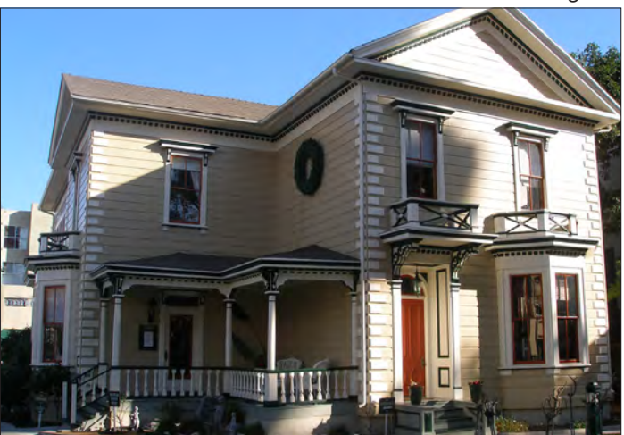
Illustrative Photo: Duplex with Porch Frontage
