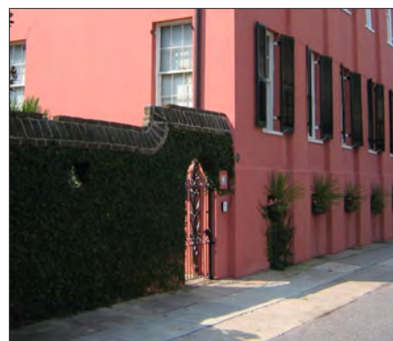
Integral 1-story wall with doorway
