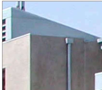
Scupper and downspout
