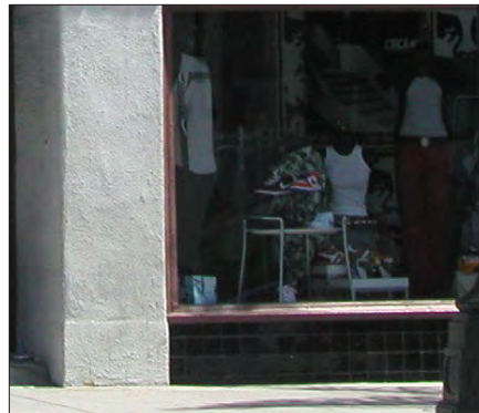
Monolithic wall and base
