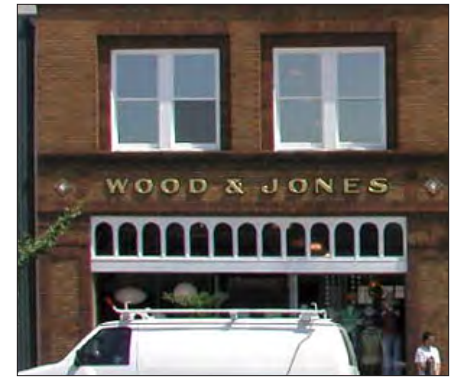
Articulated parapet with integrated signage
