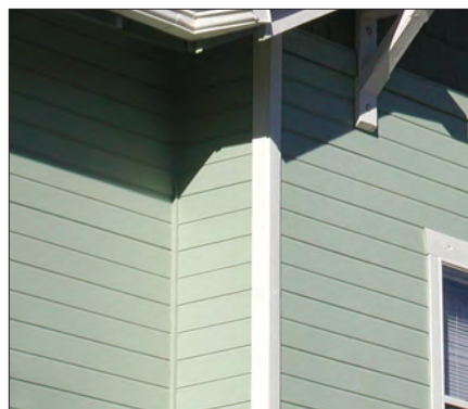
Painted horizontal wood siding
