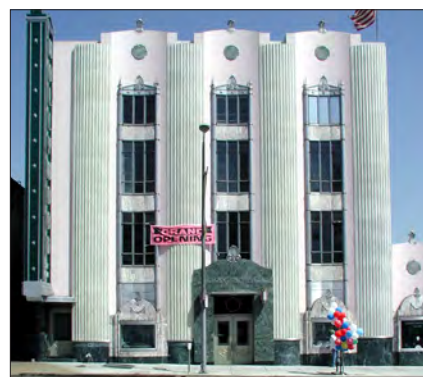
Plaster and metal
