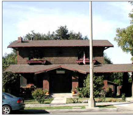
Roofs parallel to street
